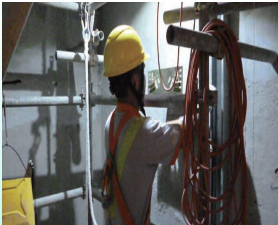
全身式安全帶要掛在升降機槽內的救生繩 Safety harness attached to lifeline inside lift shaft
